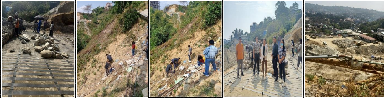
Photo: Gabion wall construction site
